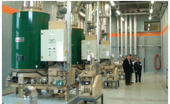
Multi unit installation of Clayton high efficiency boilers. Photo courtesy of Clayton Industries
