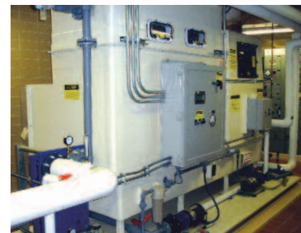
An installed liquid desiccant system. Photo courtesy of Kathabar, Inc.
