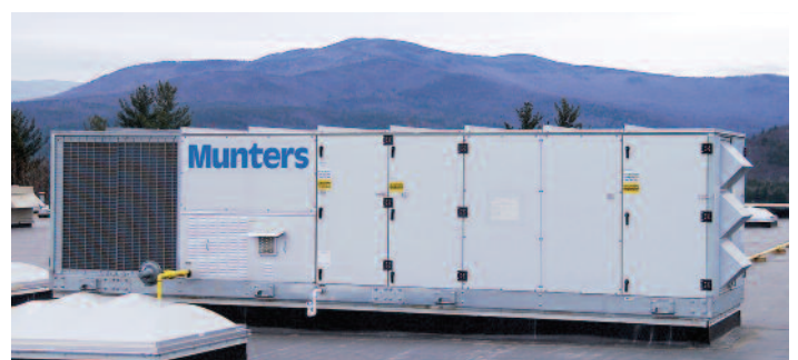
Rooftop desiccant system. Photo courtesy of Munters Corp.
